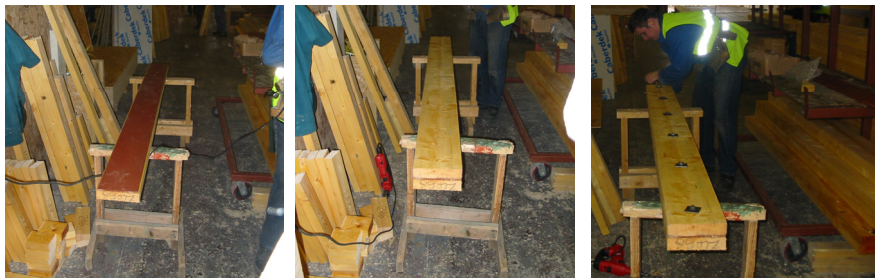
Fabrication of a bolted fitch beam
