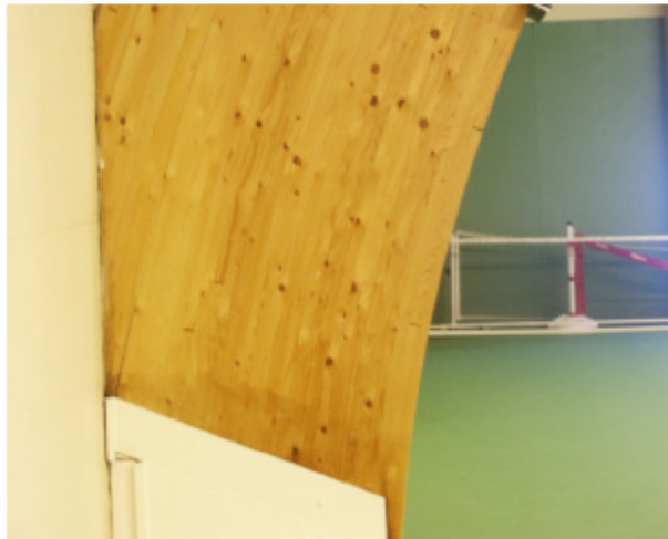
Figure 115-1. Arched column with steel parts (in white).
