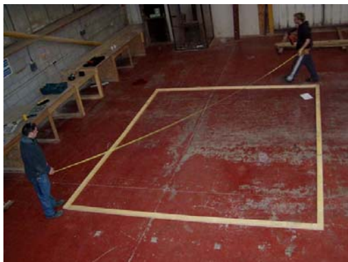
(a) A timber frame was fixed to the concrete floor using nails.
