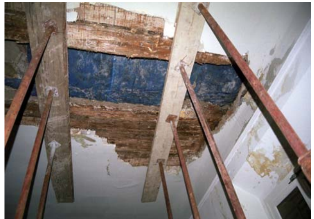
Figures 19, 20: Wetting of floor beams and failed floor
