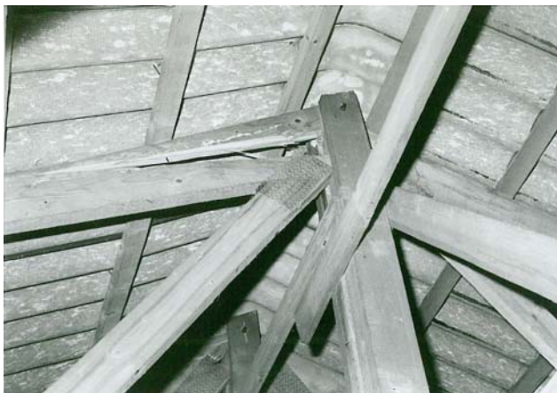
Figures 9, 10: Failure details of roof trusses connected with nail plates
