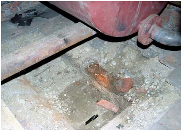
Figures 19, 20: Wetting of floor beams and failed floor
