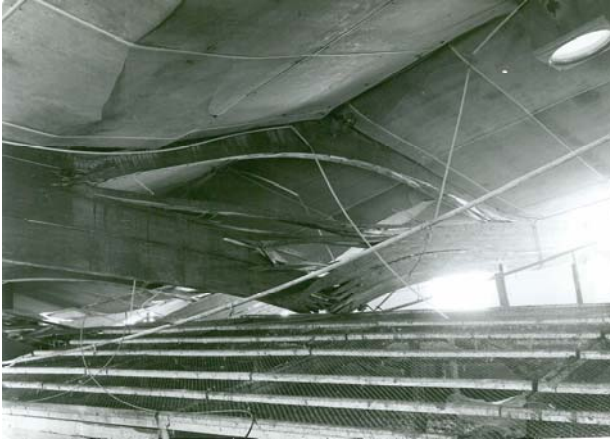
Figures 1, 2: Failed and cracked curved and tapered beams
