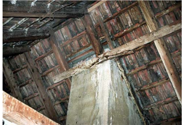
Figures 17, 18: Typical wetting points of roof structures
