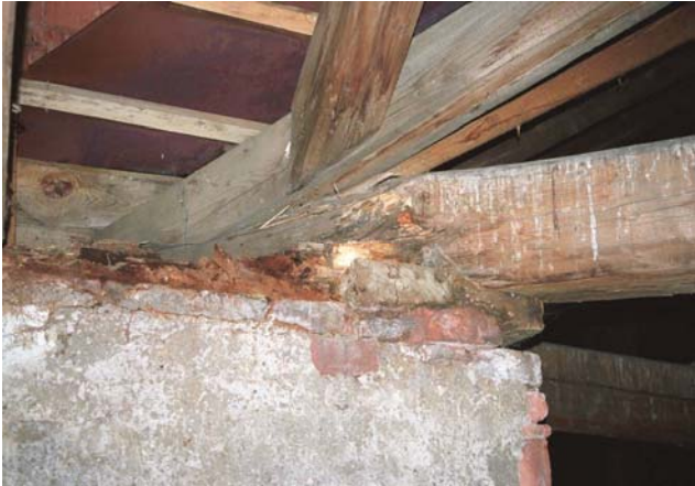
Figures 17, 18: Typical wetting points of roof structures
