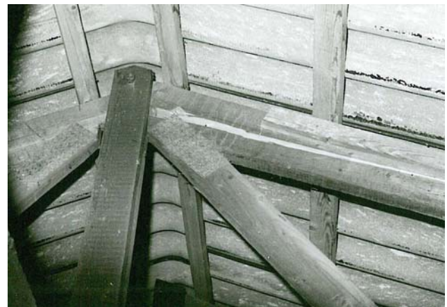
Figures 9, 10: Failure details of roof trusses connected with nail plates
