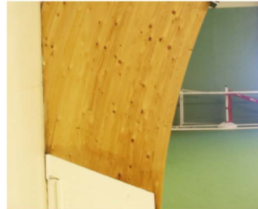
Figure 115-1. Arched column with steel parts (in white).
